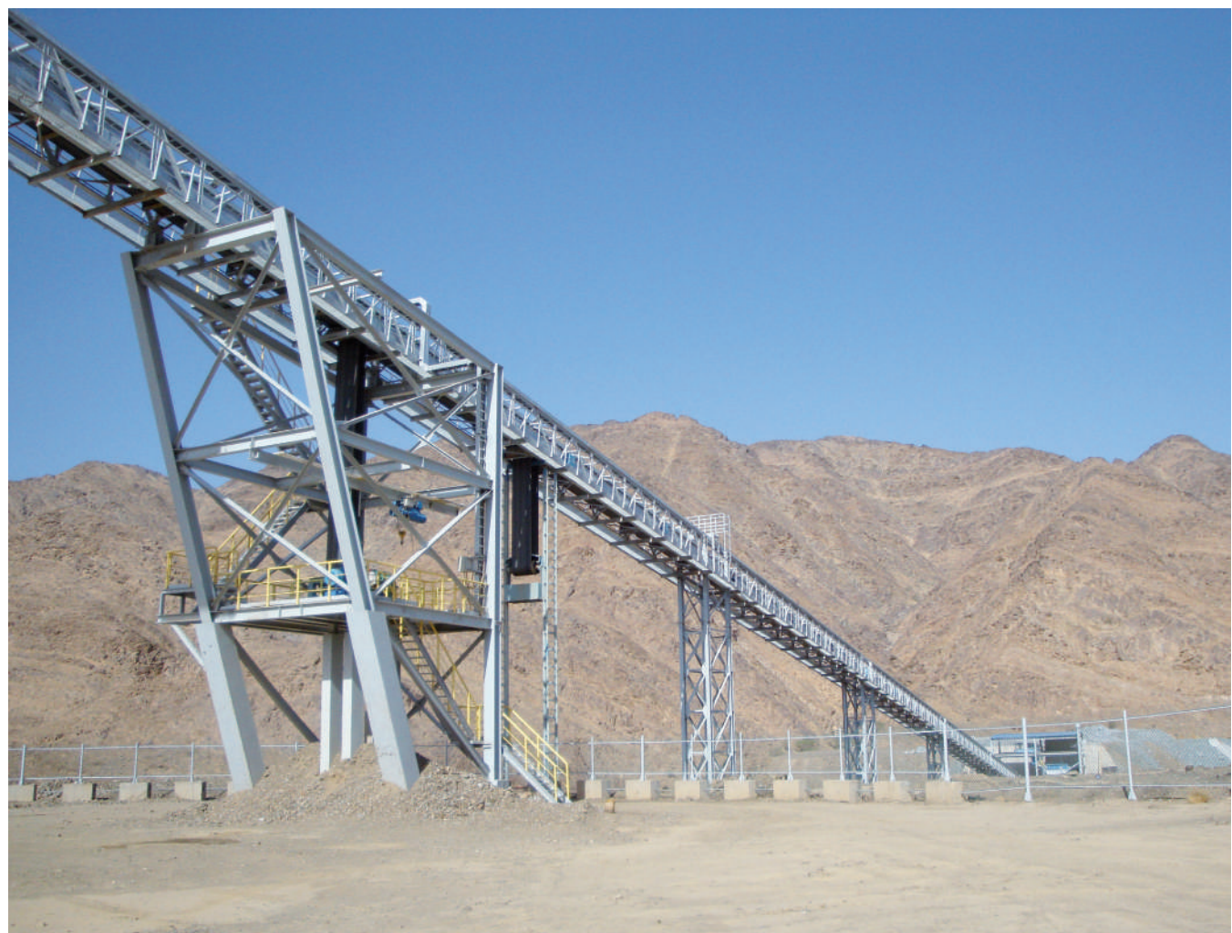
Belt Conveyor to transfer raw material from mines to plant - Al Masane Al Kobra Mining Co. / Saudi Arabia
